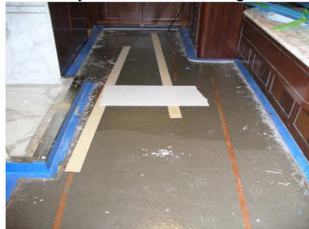
Floor-leveling polyurethane insulation ready to host the heating net
