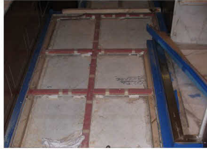
Preparation of the floor with thermo-insulating leveling resin
