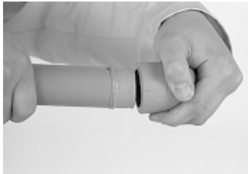
Quickly insert pipe into the fitting
