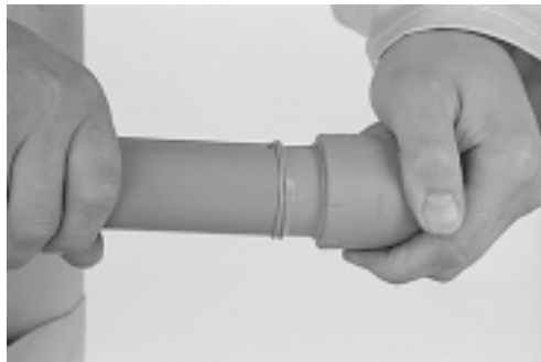
Push together without twisting
