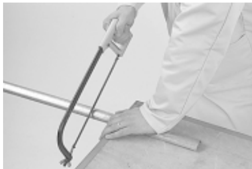
Cut to length with hacksaw
