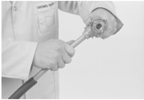
Insert the pipe into the fitting
