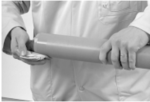
Apply cleaning fluid to cloth
