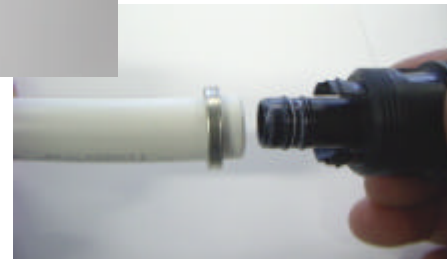
3. Replace the pipe
