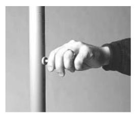
**3.** Joint the two parts and keep the repairing part for a while until cool.
