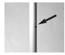
**1.** As first, adequate the hole to the hole memder dimension. They are available in 7 mm and 11 mm, respectively repairing an hole of 6 mm and 10 mm. Take the hole to this dimensions.
